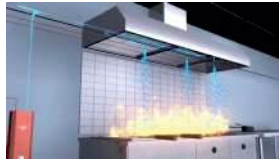
Kitchen Fire Suppression System
