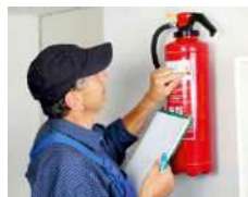
AMC of Fire Extinguishers
